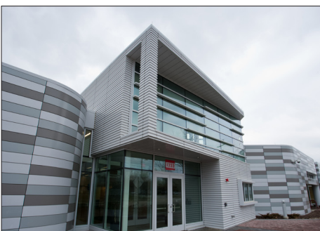
COTA Fields Avenue Bus Maintenance Facility
