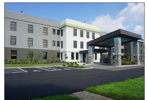
RiverVista Behavioral Health Renovation
